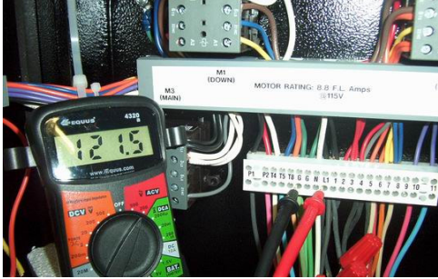
Figure 5: Proper Use of Volt meter
