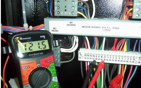
Figure 5: Proper Use of Volt meter
